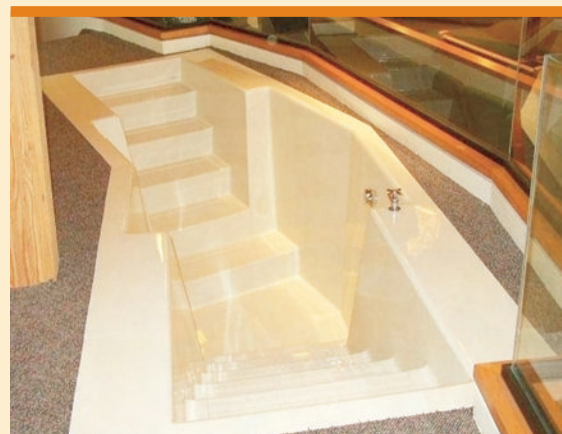
The above baptistry is a good example of providing a carpeted surface around the tank to reduce slips and falls as individuals enter and exit the tank. However, this tank still poses a slip and fall hazard as there are no handrails for the steps leading into the baptistry.
